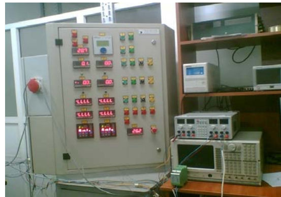
Figure 3 – Electronic control and data acquisition block
