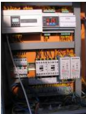
Fig.8. The electric and automation board (IHP).
