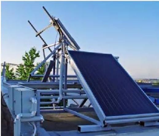
Fig. 3. Flat plate solar heat collector
