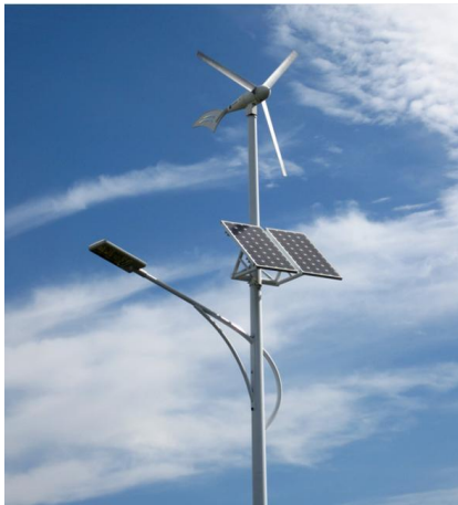
Fig. 6. Wind and solar combined system to support and power a street light
