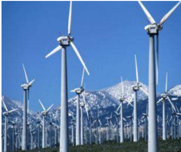
Fig. 2. Wind farm in California during winter [5]
