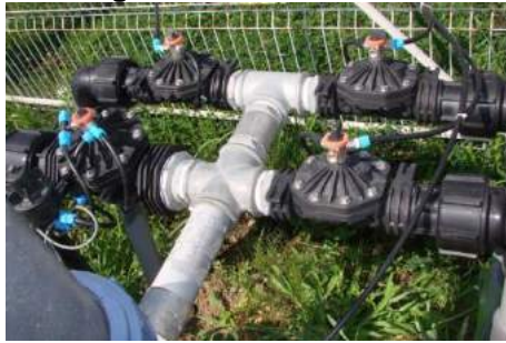
Fig. 7. Solenoid valves for irrigation plot selection
