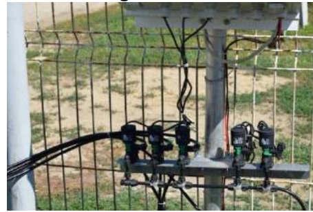
Fig. 7. Solenoid valves for irrigation plot selection
