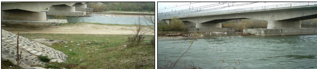
Fig. 1. Driveway bridge on DN7 at km.376+818 Strei River left - upstream view, right - downstream view
