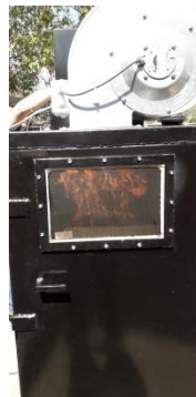
Fig. 6. Heat exchanger fan with a flow rate of 2000 m 3 / h
