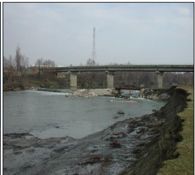
Fig. 3-left Geometrical and hydraulic characteristics of the bridge structure; -right Downstream view of the modelled concrete road bridge presenting the general scouring of the left side upper bed as produced by 2005 spring hydrological events
