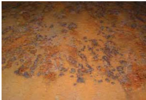
Fig. 2. Corrosion on hull plate
