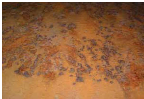
Fig. 2. Corrosion on hull plate
