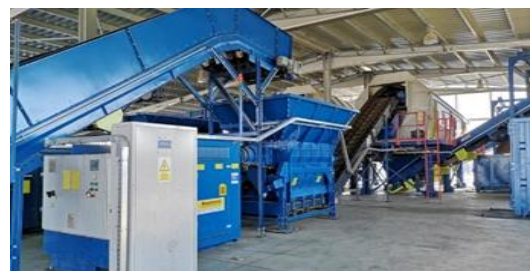
Fig. 3. Biological waste treatment station [11]
