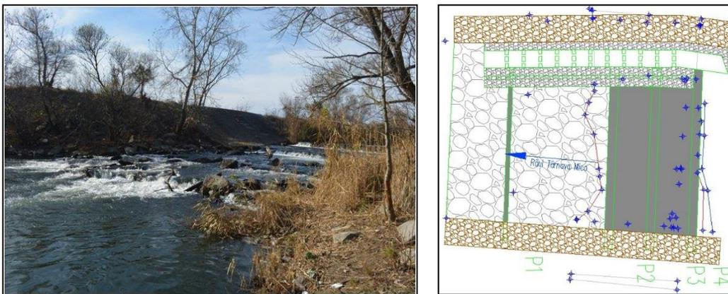
Fig. 1. Site view of the triple stepped sector on Târnava Mică River and the designed bank-view for the refurbished hydraulic arrangement with fish passage on the right bank
