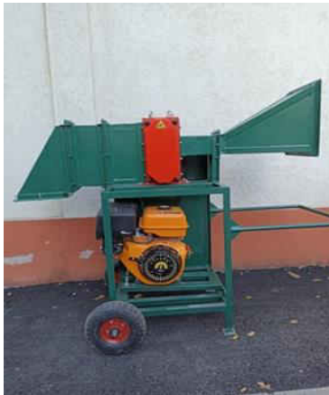
Fig. 2. Chopper driven with thermal engine of 13 CP
