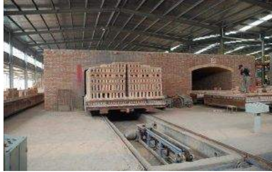
Fig. 8. Tunnel kiln for brick firing [8]
