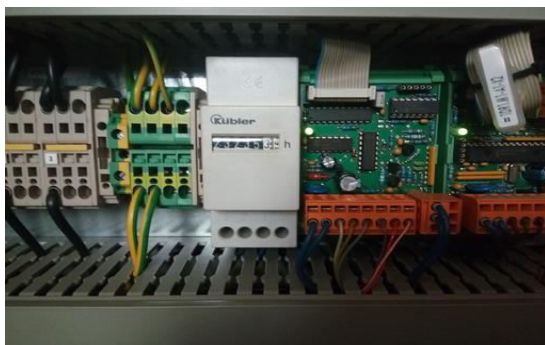
Fig. 3. Counter for the operating hours number
