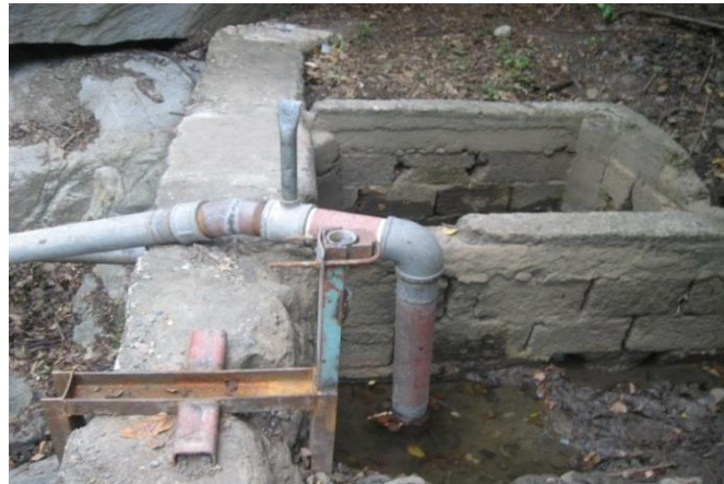
Fig. 1. Reservoir for feeding the ram
