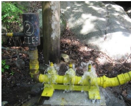
Fig. 3. 0.016 m 3 air chamber
