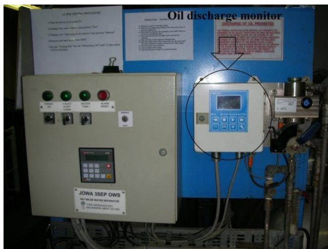
Fig. 6. JOWA type separator control panel together with PPM meter
